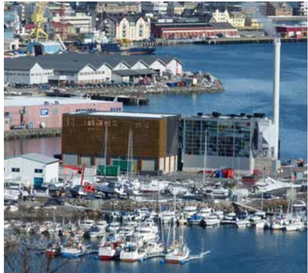
The Harstad heat plant was inaugurated in 2012 and is located in the harbor of the city.
