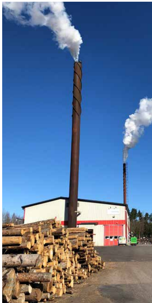
Many heat plants have storage of fuelwood ready to be chipped, to safeguard against disturbances in fuel supply, or high heat demand during exceptionally cold winters.
