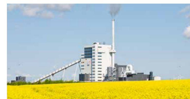
Commissioned in 2014, Kraftringen's SEK 1.8 billion Örtofta biomass-fired combined heat and power (CHP) plant is one of the largest in southern Sweden. On an annual basis the plant uses 310 000 tonnes of woody biomass to supply 500 GWh of district heat to Lund, Lomma och Eslöv and 220 GWh of electricity (photo courtesy Christina Fröjd, Kraftringen).
