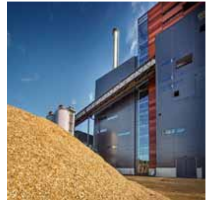
The Igelsta CHP in Södertälje just south of Stockholm is Sweden's largest CHP using wood chips. The plant produces 550 GWh electricity per year.
