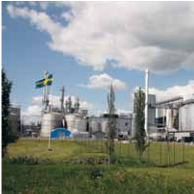
The ethanol plant in Norrköping is Sweden's largest biofuel industry.
