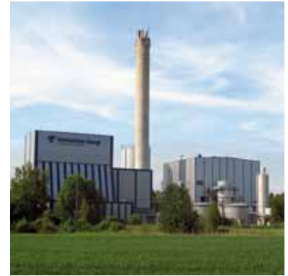
Most middle size cities now have combined heat and power plants (CHP) using biomass. This is the plant in Katrineholm west of Stockholm.
