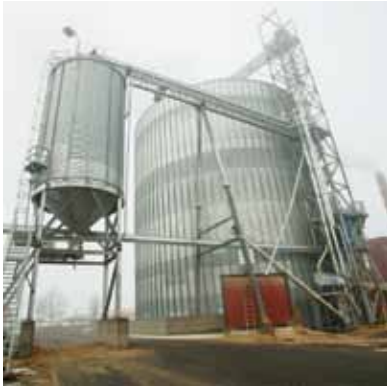
Pellets are produced from sawdust and shavings in 80 factories around Sweden. The picture shows the pellet storage silo at Derome.
