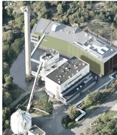
GoBiGas Phase 1 20 MW bio-methane Demonstration Plant
