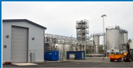
St1 refinery in Gothenburg; Etanolix® unit.
